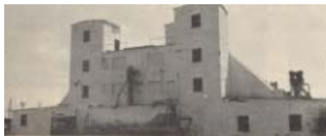
Ill. 24. Hill County Cotton Oil Co., south side of W. Franklin and west of railroad tracks. Built 1917.
