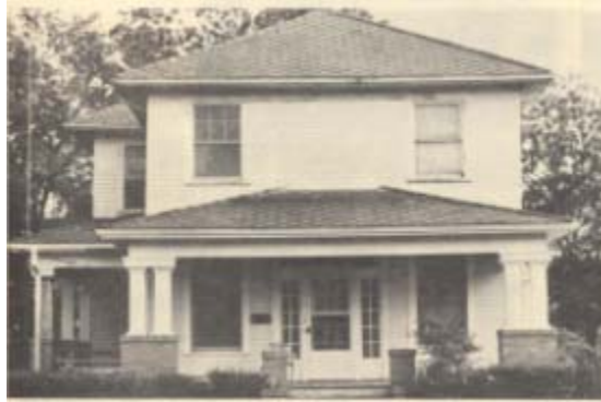
Ill. 19. 400 E. Franklin. An earlier house on the lot burned, and this variation of the four-square house was built circa 1925.
