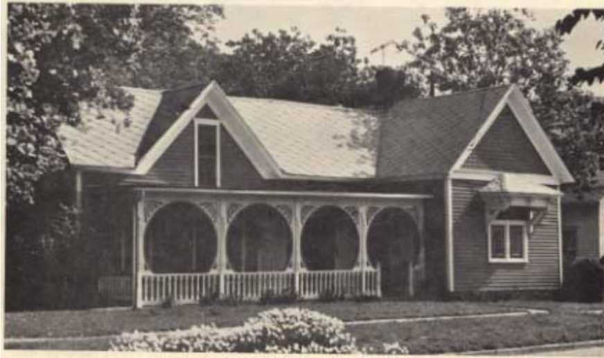
Ill. 6. Liner-Rhoads House, 315 Corsicana. Built circa 1885.
