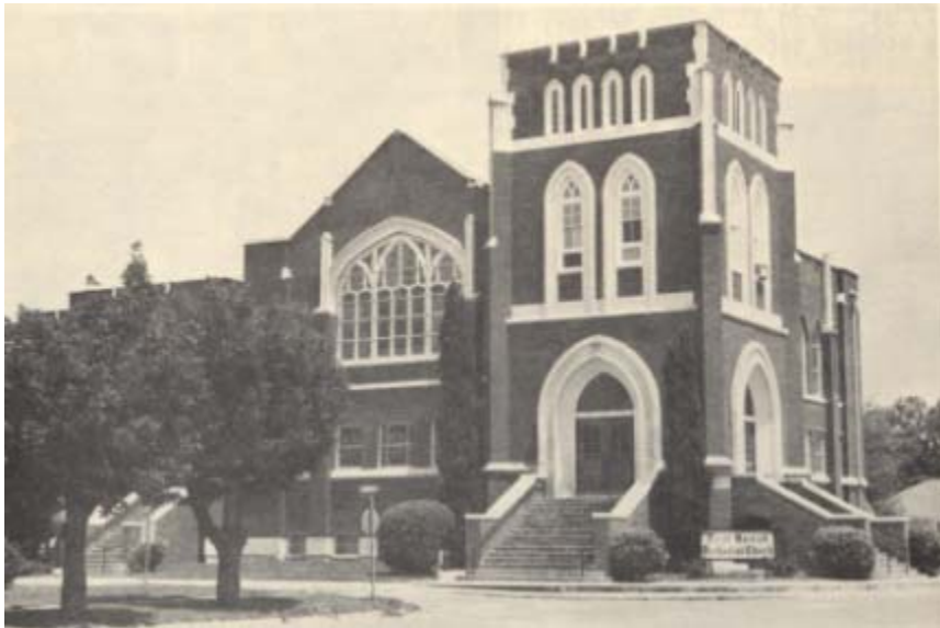
Ill.32. First United Methodist Church, 315 E. Elm. Originally built in 1914 and burnt and rebuilt in 1928-29.
