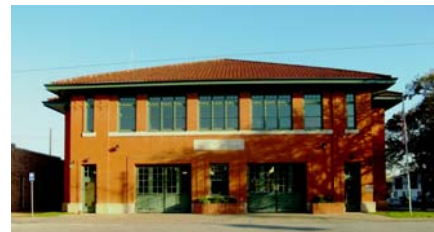
Historic City Hall: 127 E. Franklin Built in 1909-1910 by Tom Sowell, contractor/builder.
