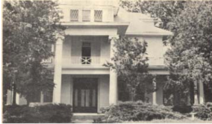
Ill. 21. Satterfield House, 311 Craig. Original house built in 1895, and enlarged in 1906-08. An example of the Classical Revival Style in Hillsboro.
